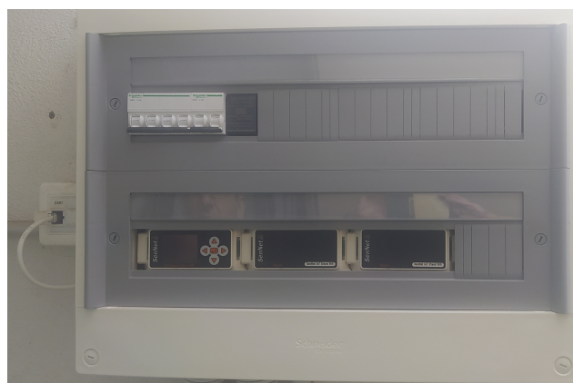
Figure 5. Sennet IoT DL271 Datalogger Long Net (the first device on the left) and 2 Sennet IoT Xtend M6.
